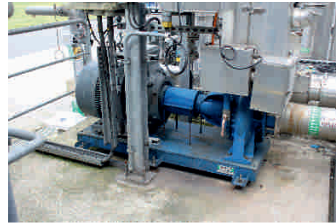
Series NT150-400/02, capacity 350 m 3 /h, 5 bar, liquid cooling water, process: cooling water system.
